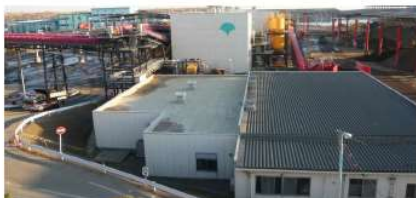
Main Building of Tokyo Metropolitan Construction Waste Soil Recycling Center (Source: Center's Website)
